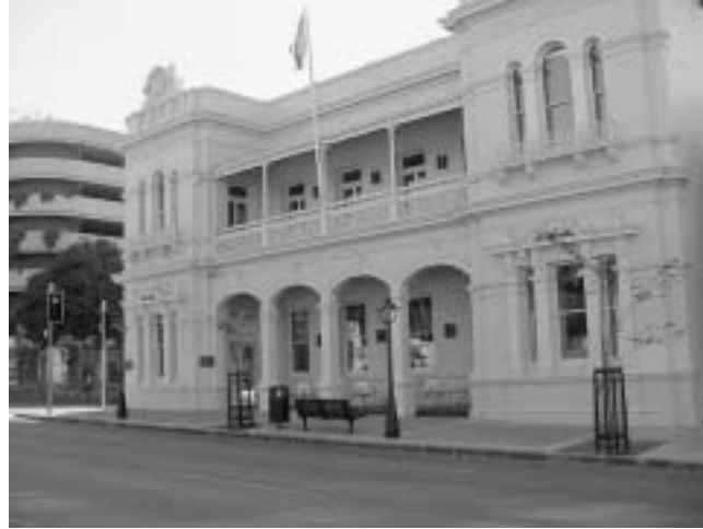
Figure 1: External view of main section of the refurbished post office (Photography: Author)
