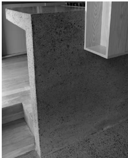
Figure 2: Folded concrete slab.
