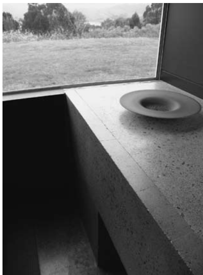
Figure 1: Ground level concrete slab
