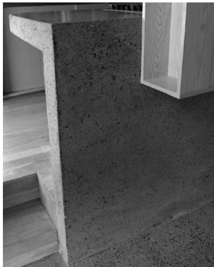
Figure 2: Folded concrete slab.
